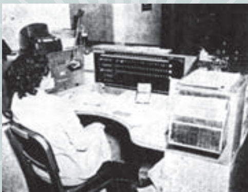
Police Switchboard and Intercom Room.
